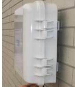
FDB fiber termination box on the pole FDB fiber termination box on the wall
